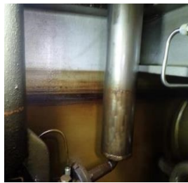
Images: Top left = varnish-covered thermostatic control valve Top right = varnish in oil reservoir head space Bottom left = varnish bathtub ring in oil reservoir Bottom right = heat exchanger cooling plate with partially removed varnish
